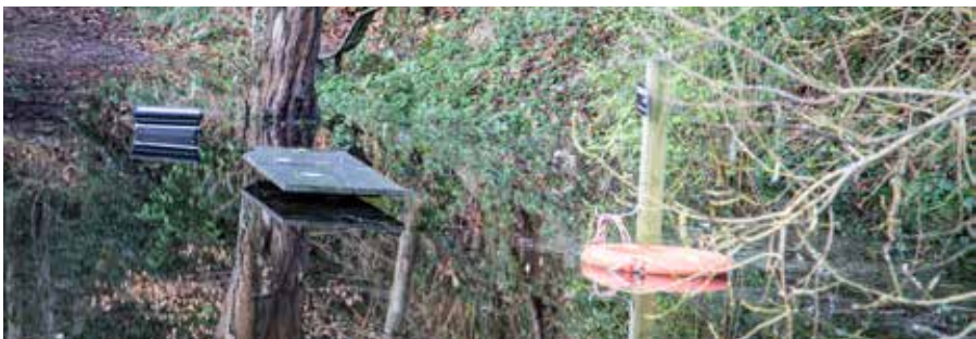
Quarry Pond litter bin and bench at the height of this year's flood
